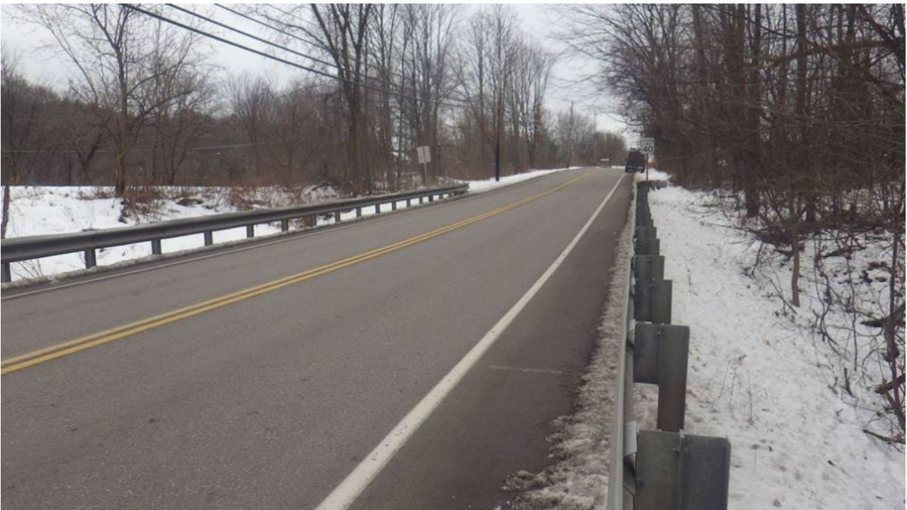
Looking South on VT Route 2A over Bridge 11 (Inspection photo 2021)
