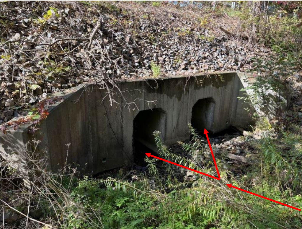
Frankenstein structure inlet from TH-24 (true inlet, first section, of 3-part structure) (red arrows show direction of flow)
