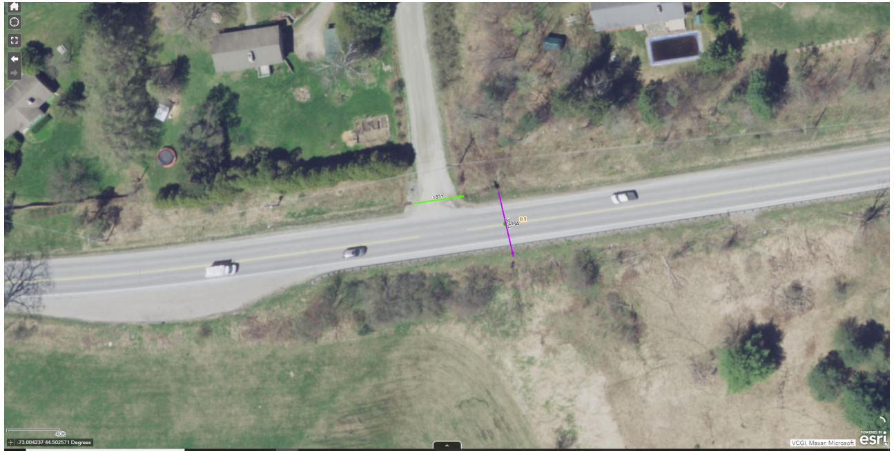
Figure 6. Bridge No. 6A, Jericho
