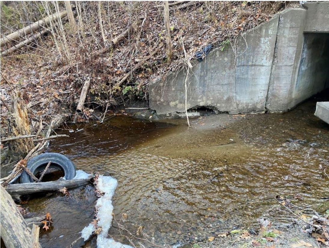
Northwest wingwall of outlet (Inspection photo 2021)
