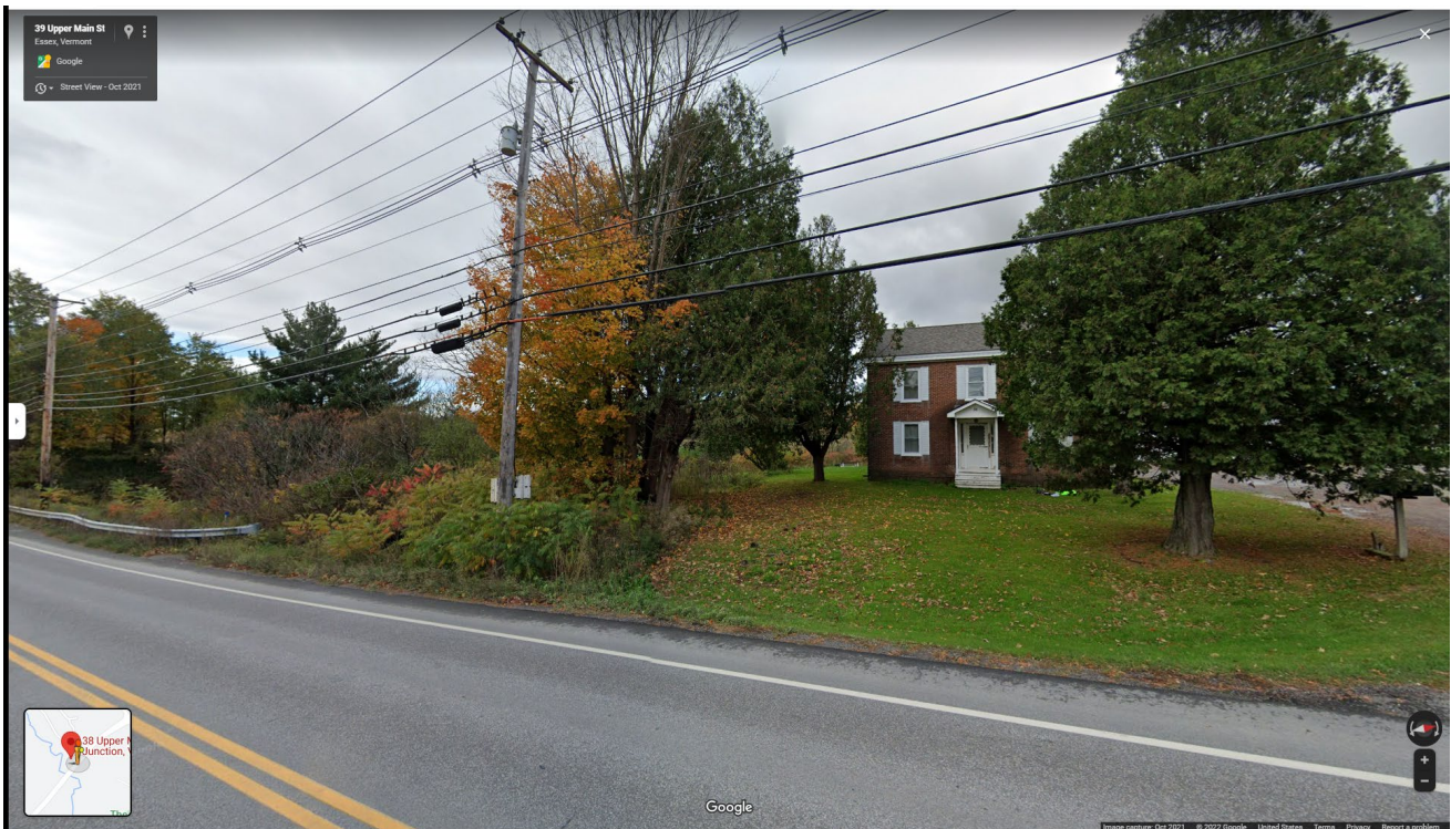
Figure 1. 38 Upper Main Street at northeastern corner of Bridge No. 2 in Essex.
