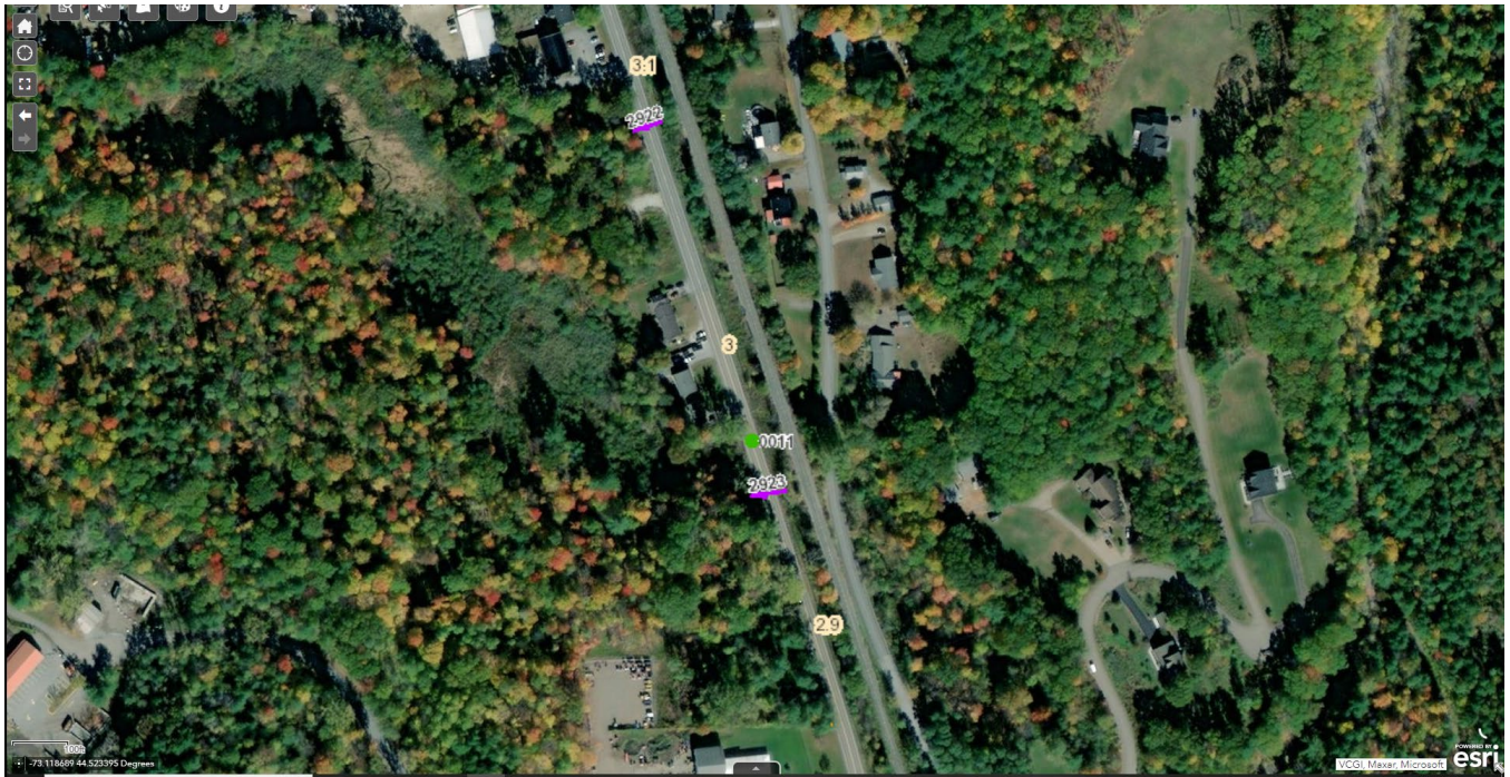
Figure 4. Bridge No. 11, Essex
