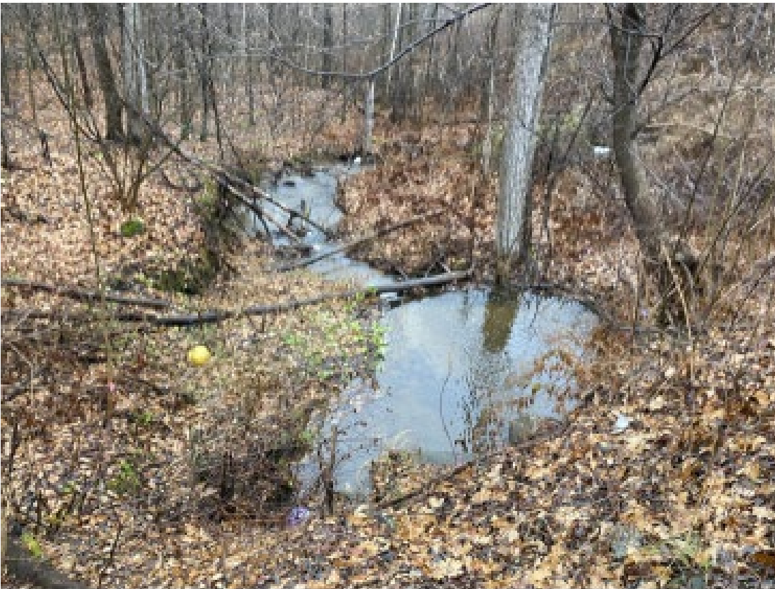
Downstream Channel (Inspection photo 11/28/2022)
