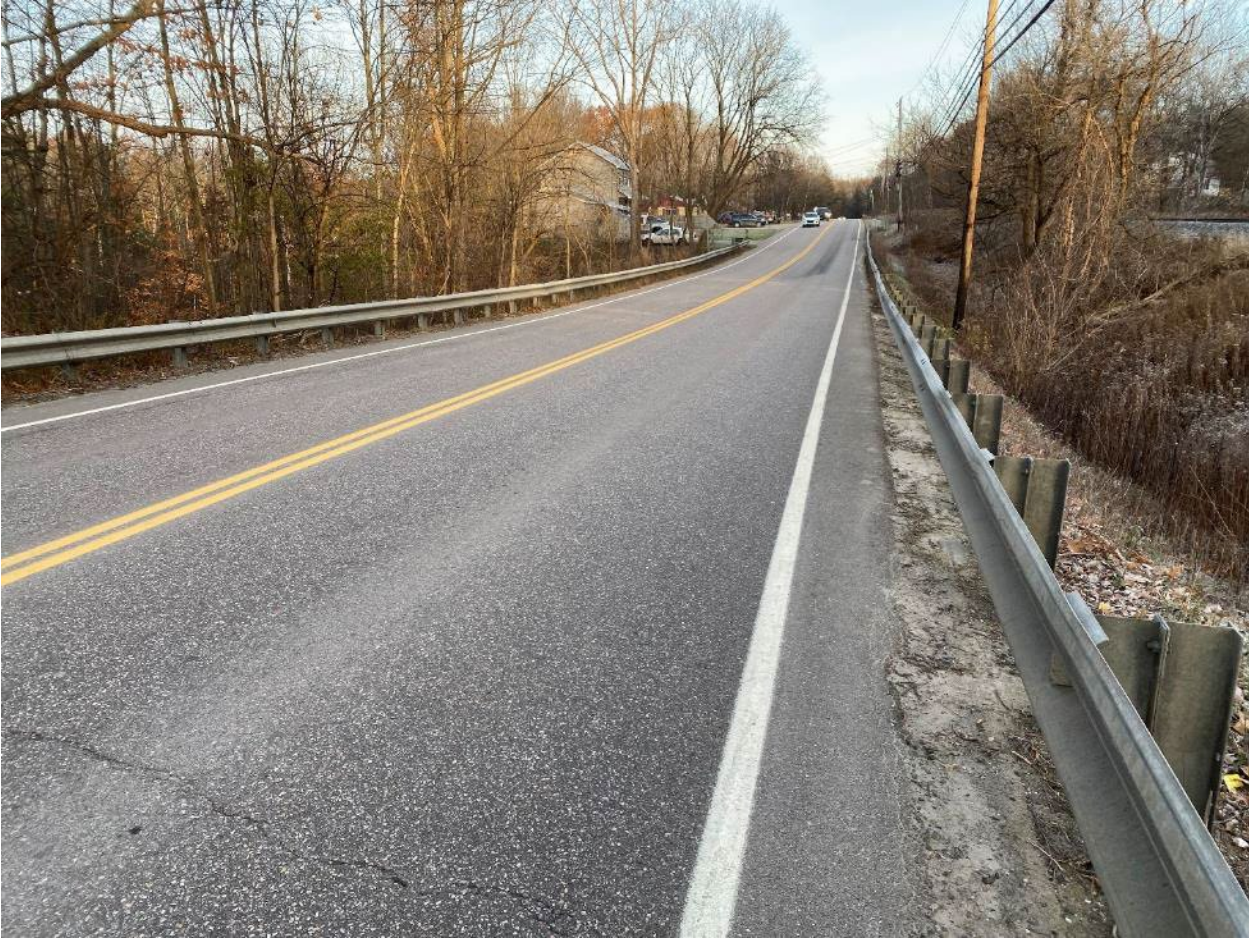
Looking North on VT Route 2A over Bridge 11 (Inspection photo 2021)
