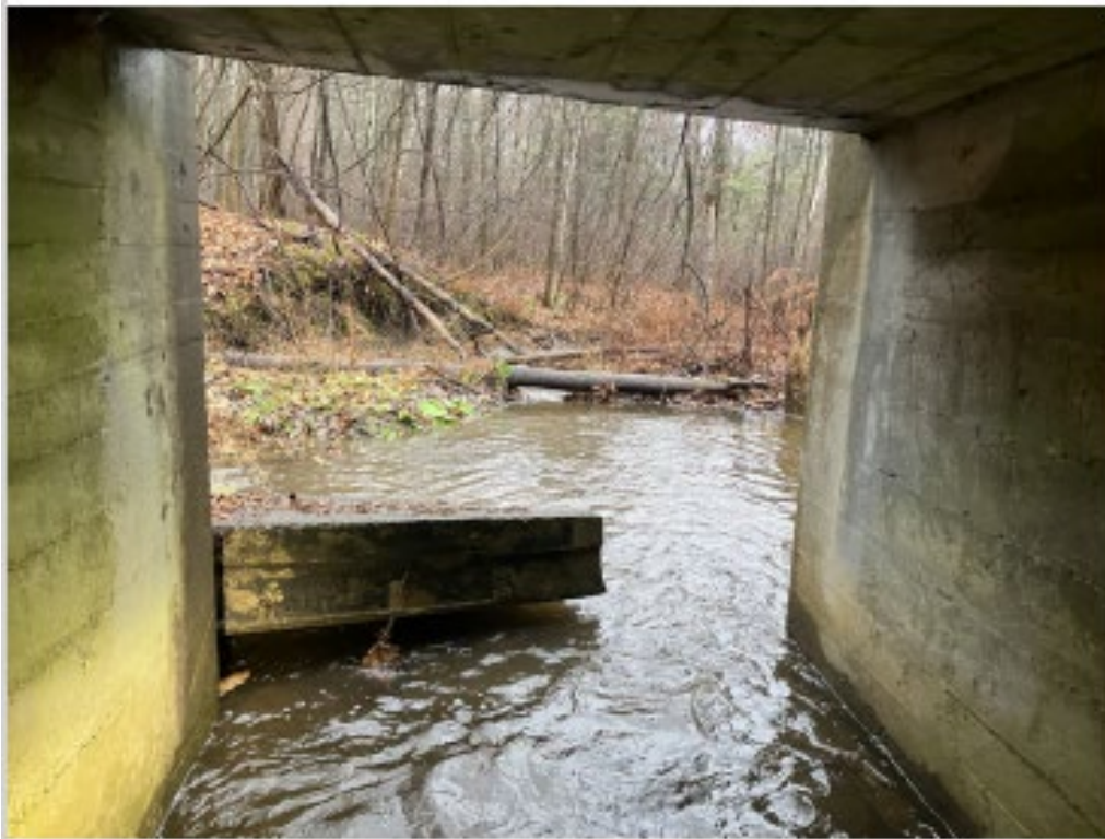
Downstream End of Culvert (Inspection photo 11/28/2022)
